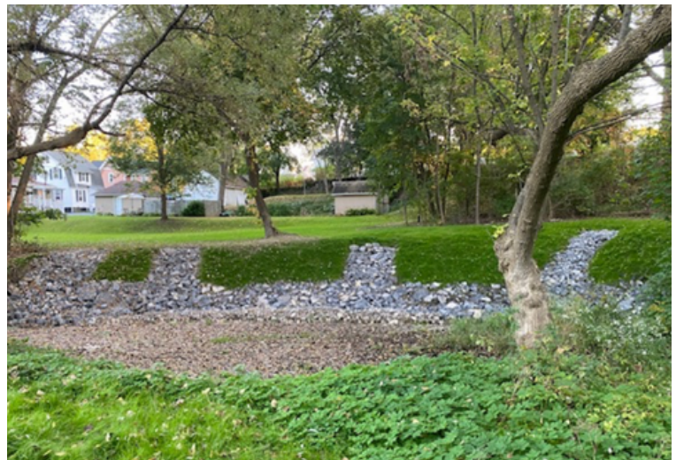
Figure 4. Boulders positioned and planted grasses stabilize the banks (October 2023)
