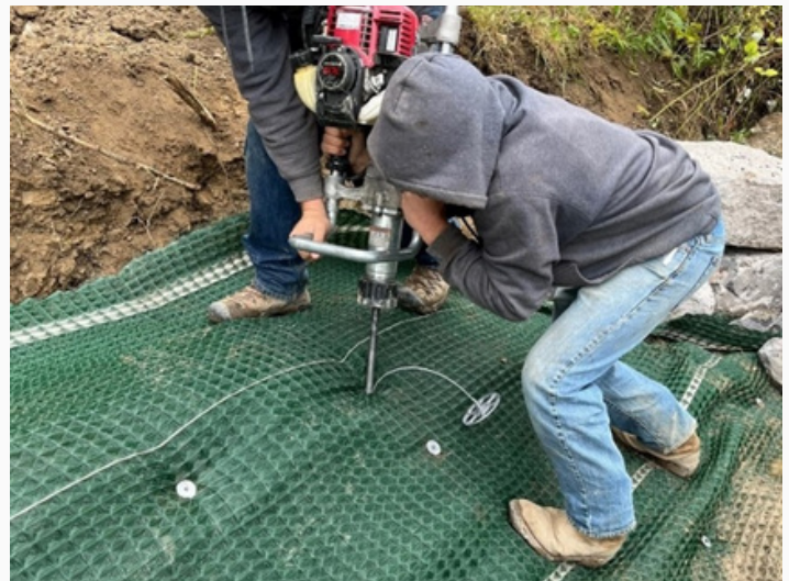
Figure 2: Armormax stabilization fabric being mechanically fastened into place in the ditch
