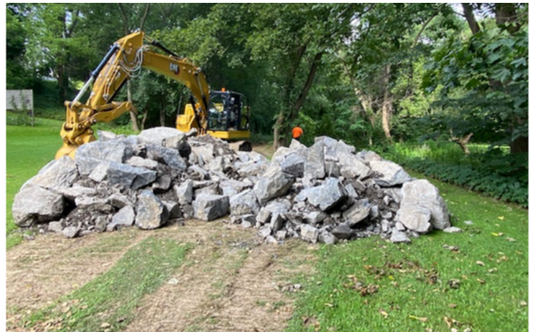
Figure 3. Boulders brought in to stabilize the stream banks
